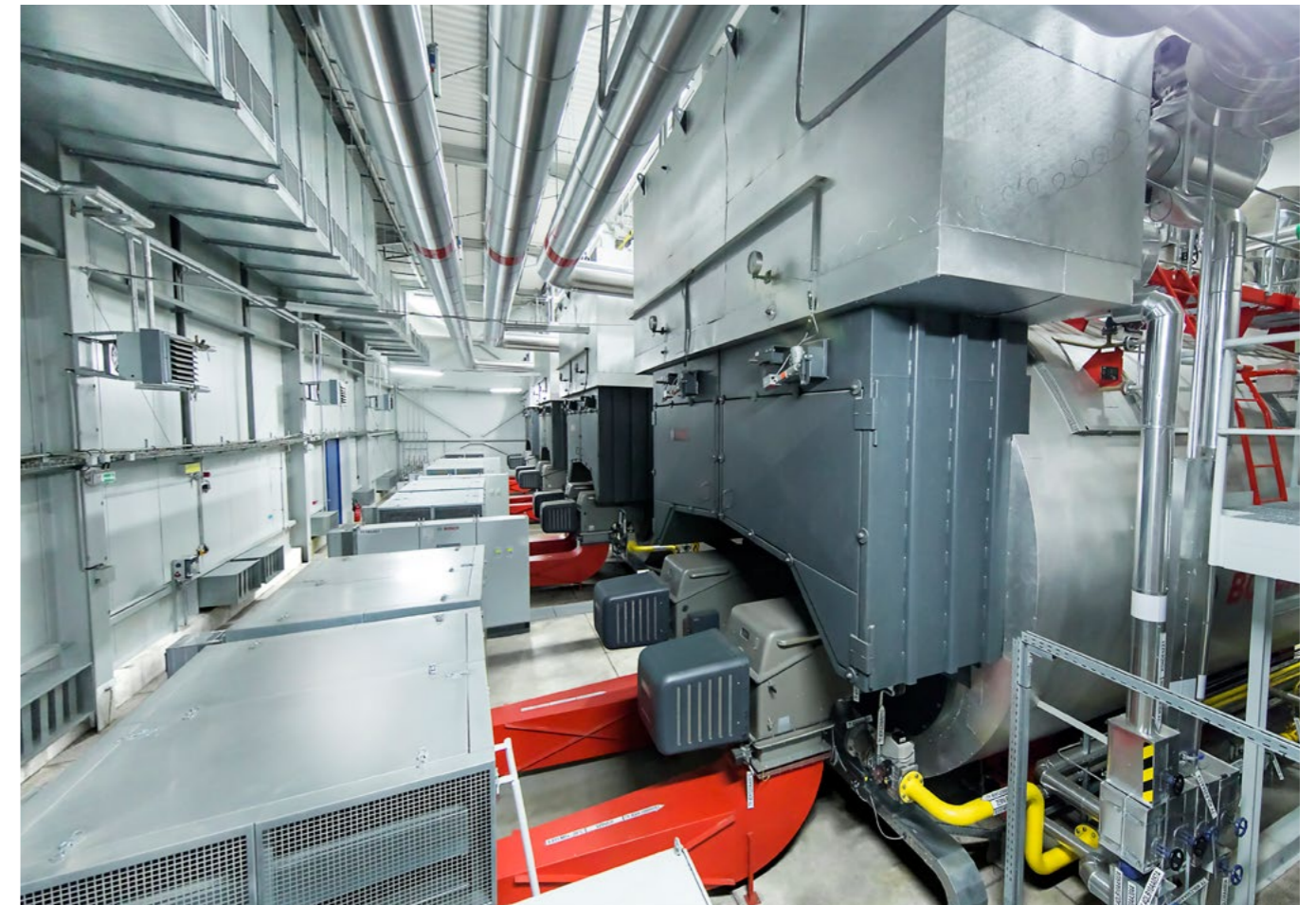
The superheater modules are installed on the front reversing chamber of the boilers.
