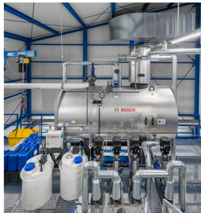
Water service module WSM
