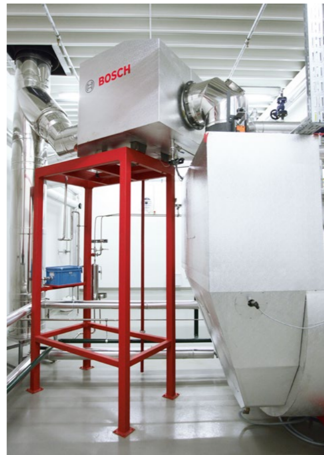
Integrated flue gas heat exchanger and flue gas heat exchanger for condensing use
