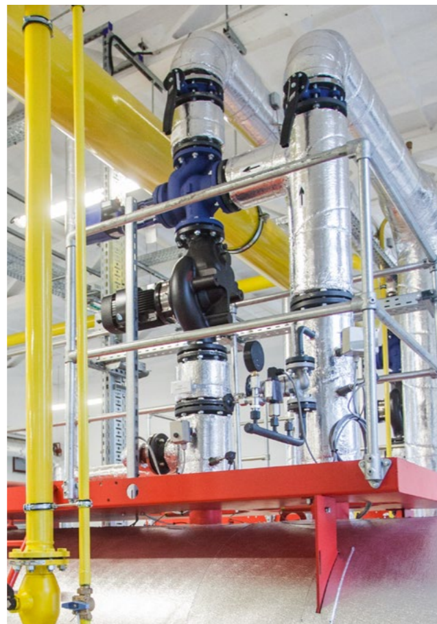
Return flow temperature safeguard RTS
