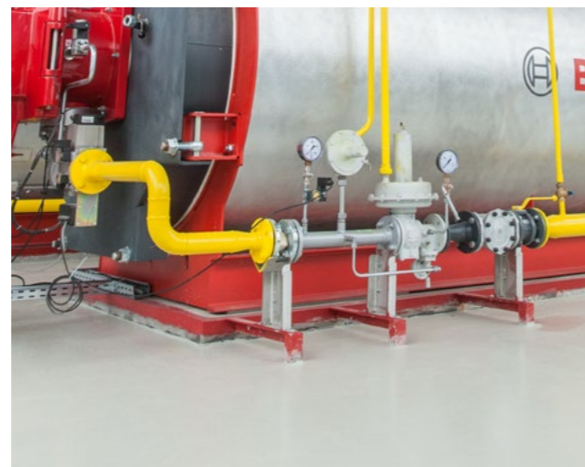
Gas regulation module GRM
